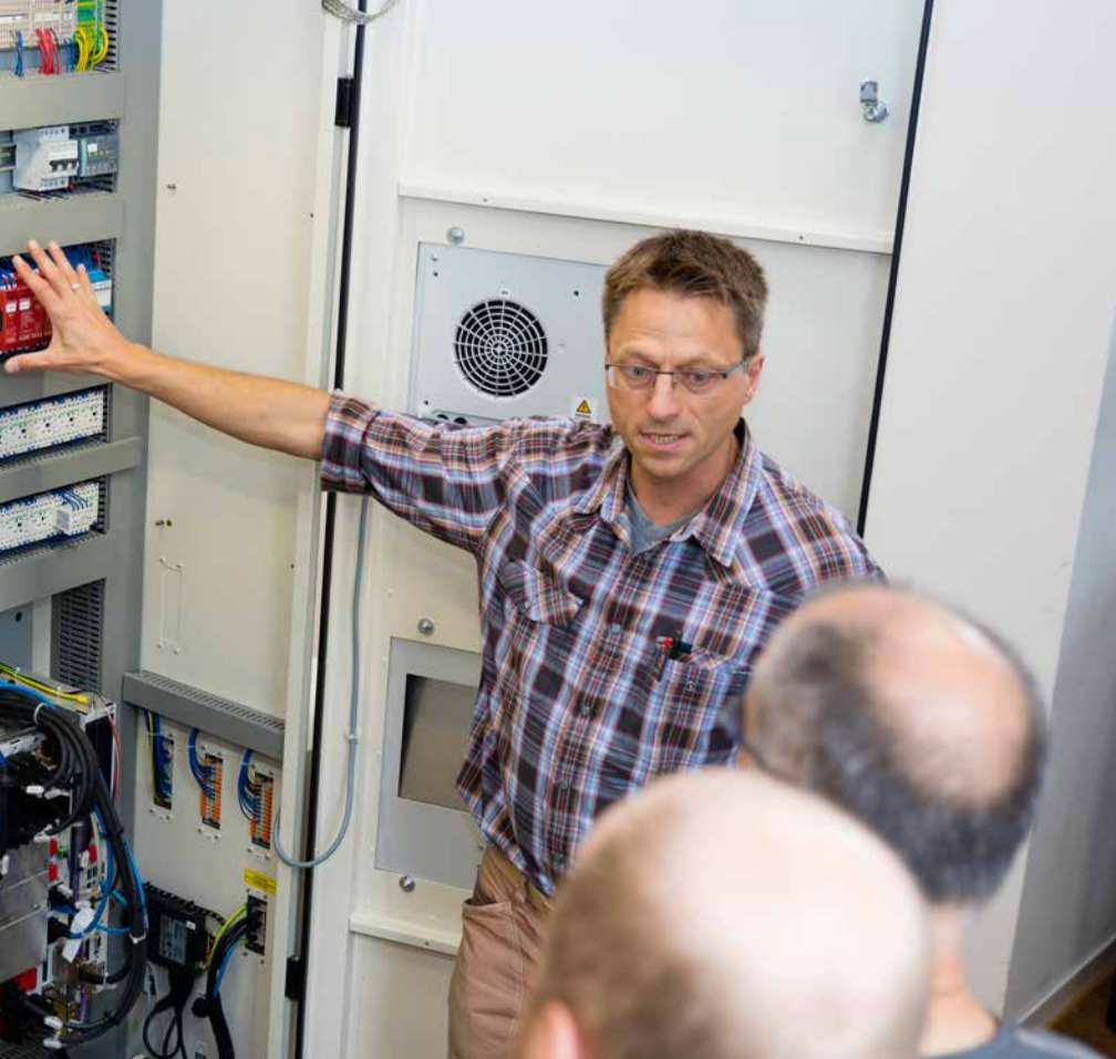
The preferential work environment in the practical section of service courses—the technology in the machine's electrical cabinet
